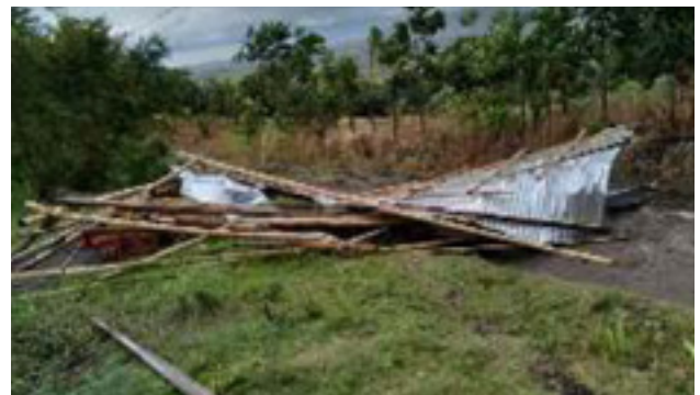
This is all that's left of one of the classrooms. There were 3 more buildings that were also demolished.
