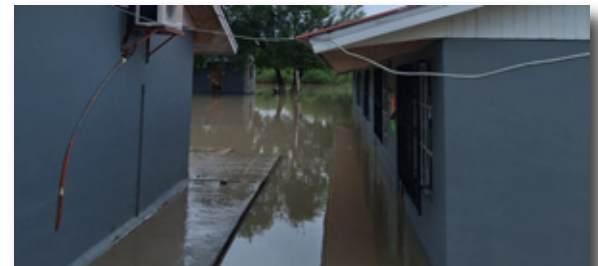
The water was several feet deep in each of the school's buildings.
